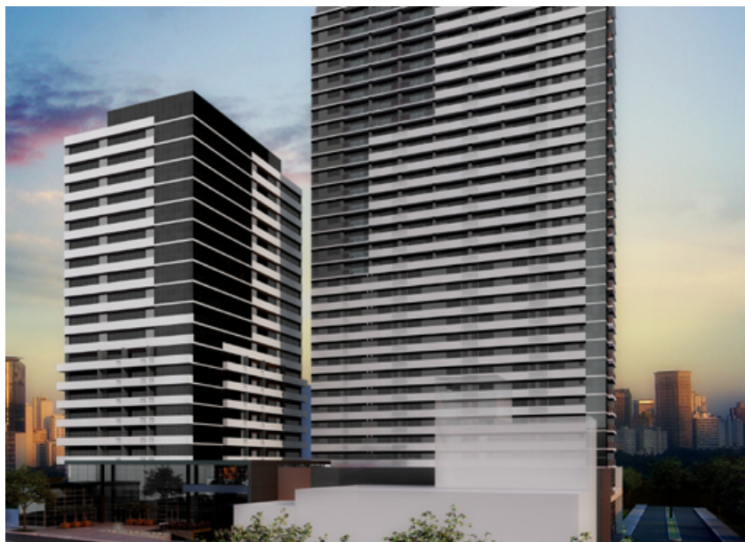
TECNISA inicia as obras do The Five – East Batel
